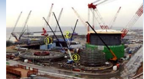
Under Construction COD TBD
