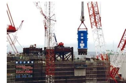
Under Construction COD TBD
