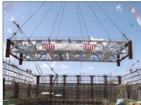
Roof Truss Steel
