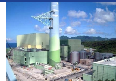
Under Construction COD 2014 (estimated)
